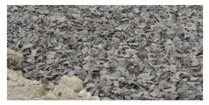
3. Completion of cell including geotextile fabric on top of tire shred (September 14<sup>th</sup>)
