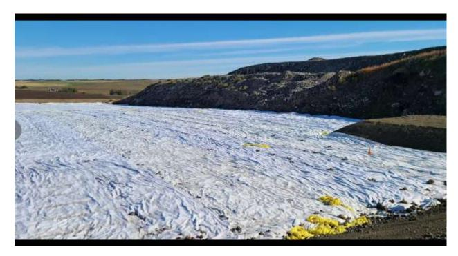
4. Early stages of placing MSW on top of liner. (September 21<sup>st</sup>)
